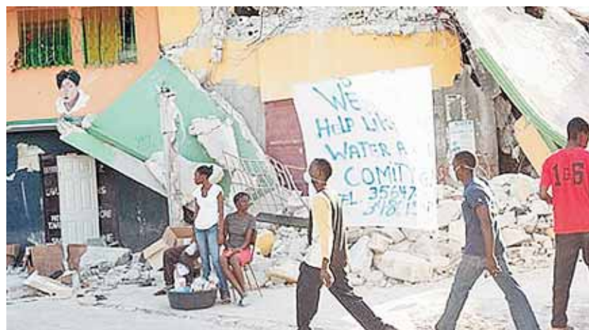
Signs requesting help are a common sight in earthquake-damaged areas in Port-au-Prince, Haiti.
