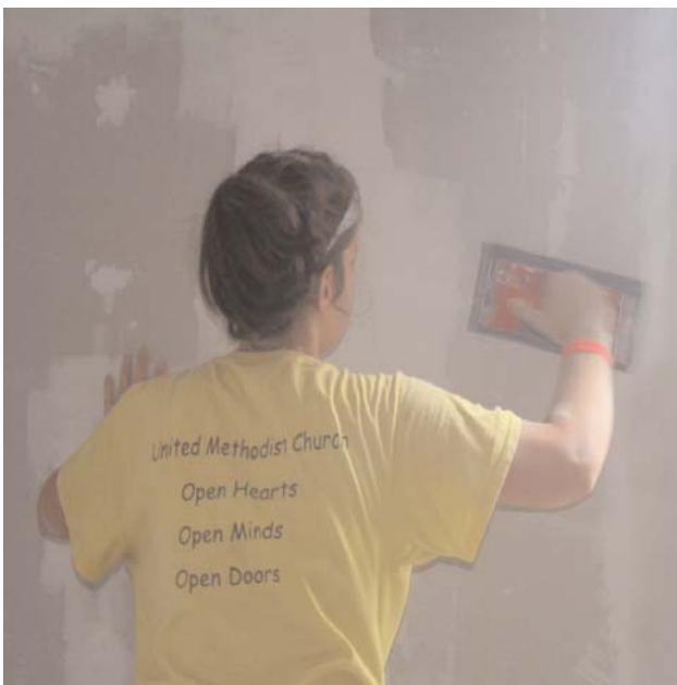
Crystal Adamson, a volunteer from Missouri perfects her sheetrock installation skills.
